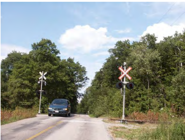
Photo 12-7: At Grade Rail Crossing with Lights only – Steeles Avenue east of Milborough Line
