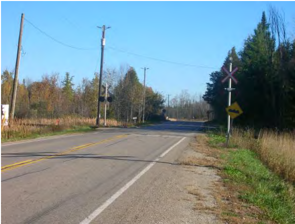
Photo 12-1: At Grade Rail Crossing with Lights only – Campbellville Road west of Twiss Road
