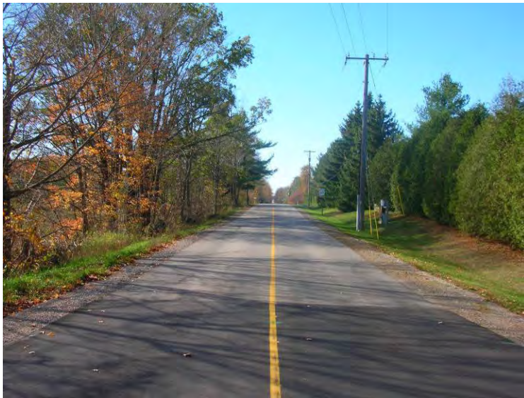
Photo 12-8: Concession 11 E west of Centre Road looking in the Westbound direction
