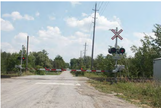
Photo 12-4: At Grade Rail Crossing with Lights and Gates – Twiss Road north of Campbellville
