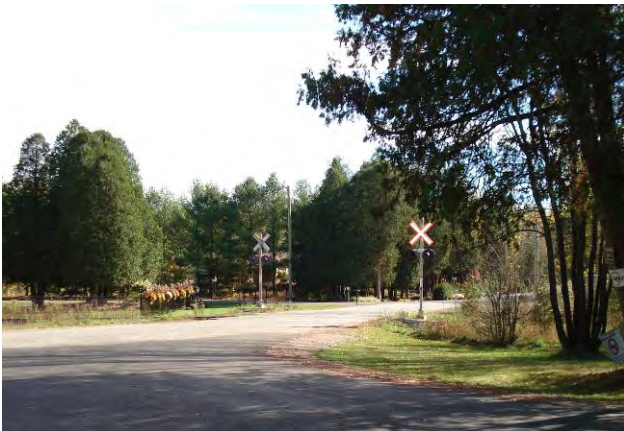
Photo 12-6: At Grade Rail Crossing with Lights only – Milborough Line just south of Concession 10E
