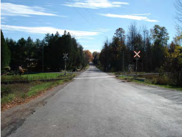
Photo 12-5: At Grade Rail Crossing with Lights only – Milborough Line north of Campbellville Road
