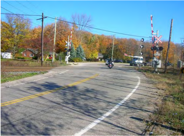
Photo 12-2: At Grade Rail Crossing with Lights and Gates - Campbellville east of Twiss Road
